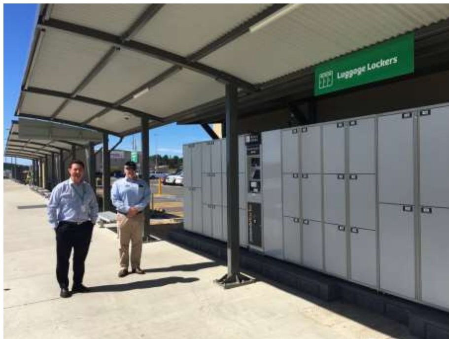
Hobart Airport car park. February 9, 2022. To promote protective clothing for commuters TAC should sponsor lockers at park & ride facilities.
